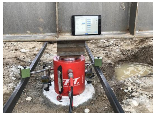
Fig. 6 App in use during pile compression test
