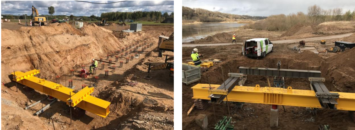
Fig. 3&4 Work site where pile load tests are conducted
