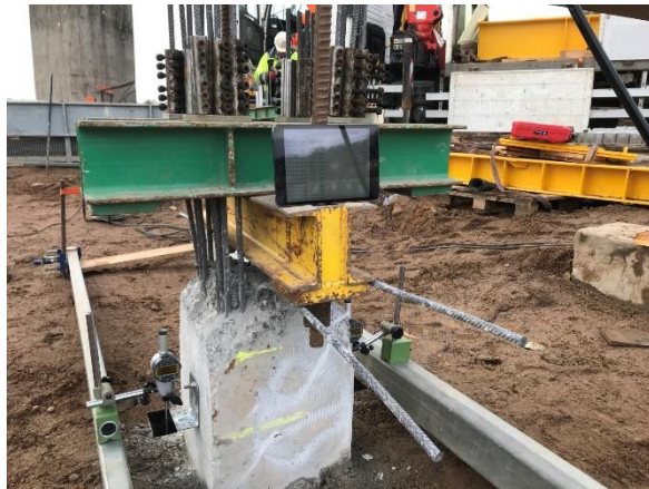
Fig. 2 Tension Load Test
